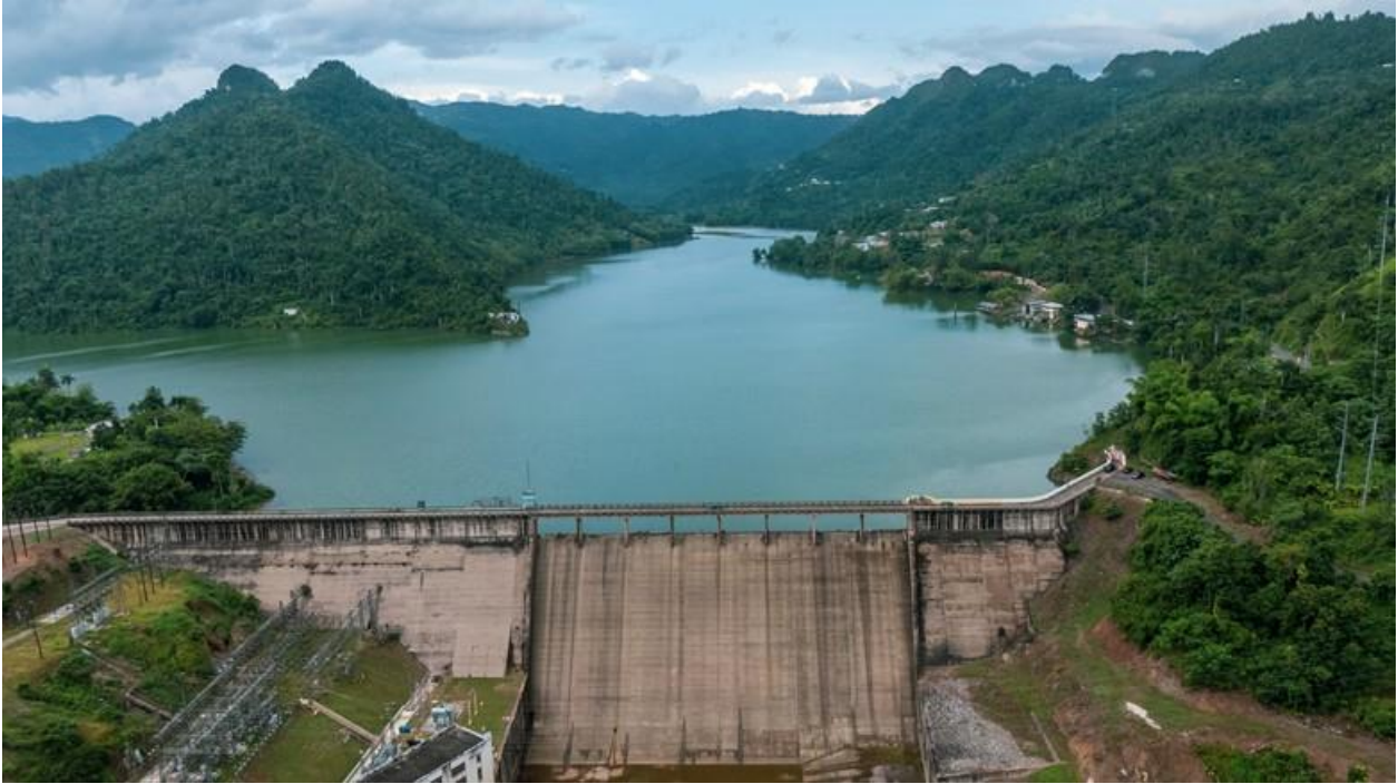
Figure 2 - Dos Bocas Hydroelectric Plant
